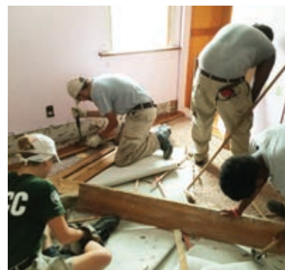
Volunteers from Ameri-corps help repair a home damaged by the tornado.
